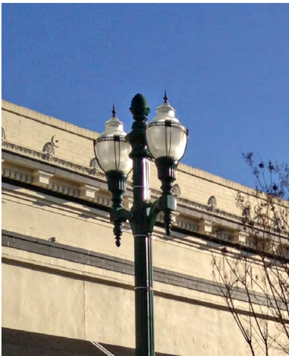
Top: Pedestrian-scale lighting on Route 16 / Main Street in Woodland helps illuminate an evening holiday street fair. Bottom: Lighting fixtures on a local road in Alameda complement local architecture.
