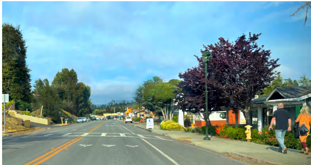
Top: On Route 299 in Willow Creek a welcome sign, street trees, and landscaping visually reinforce the transition from a higher-speed rural facility into a lower-speed rural downtown main street environment. Bottom: On Main Street in Cambria, sidewalks, pedestrian lighting, and pavement markings further signal a transition to a lower-speed environment on the approach to downtown.
