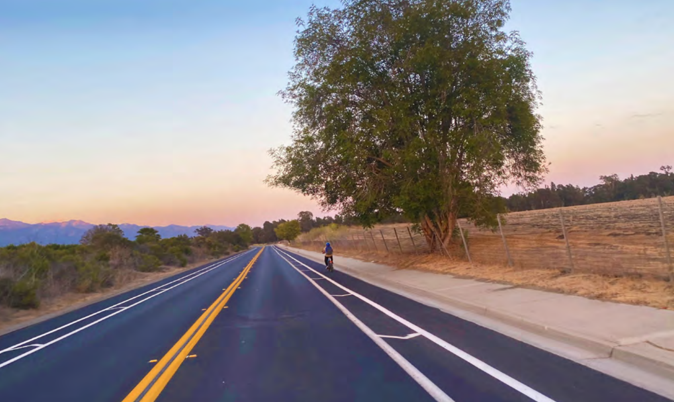
Above: A buffered bike lane on Route 135 / Bell Street in Los Alamos. Below: A buffered bike lane on a local road in Goleta.
