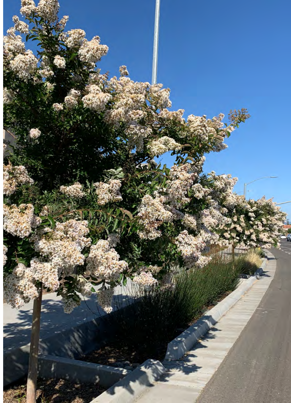
Above: A planter on a Jose city street is designed to capture storm water and contains plants that are suited for period of inundation with water.
