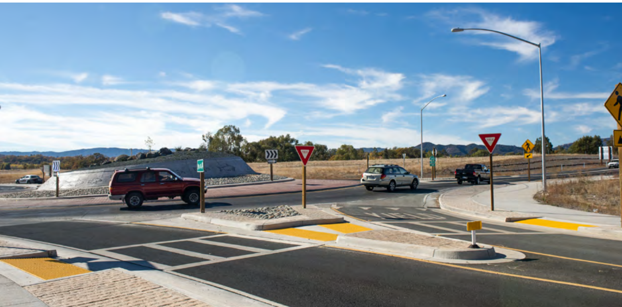
Top: A roundabout on Highway 1 south of Fort Bragg. Bottom: A roundabout in Upper Lake on Highway 20.
